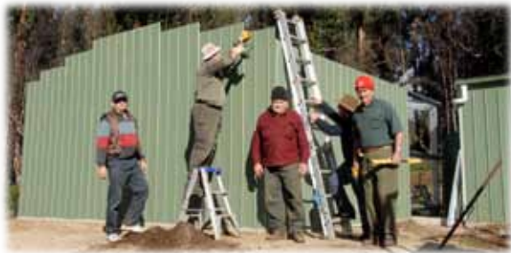
Rotarians from Broken Hill South construct a shed in Calligne to be used as temporary accommodation
