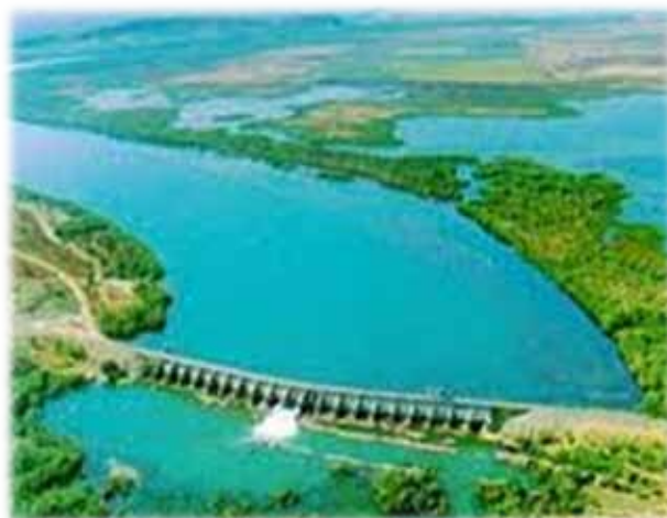
The Ord River Diversion Dam with Lake Kununurra. View looking southward
