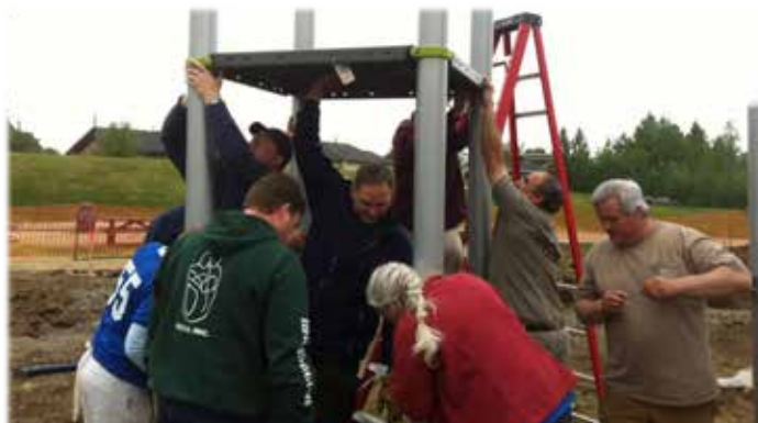
Members and local volunteers worked together to erect the playground equipment.
