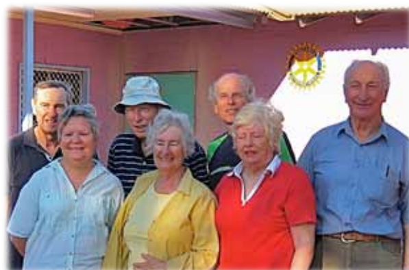
Working party engaged in completing the interior of the building outside the Purple House 2 at Kintore.
